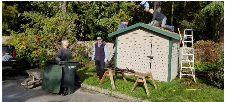
Don, Arnie, Steve and Rick give the shed a new roof
