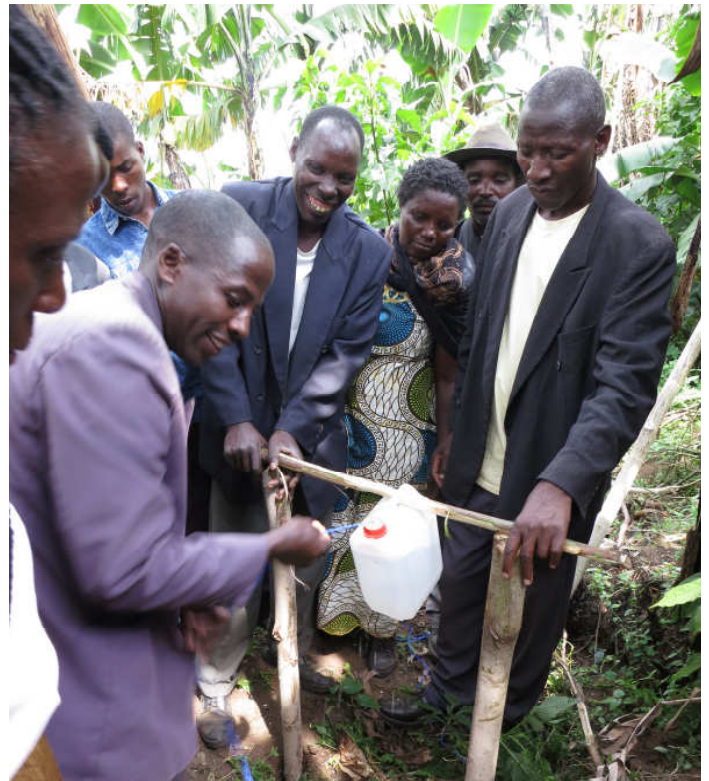
Building a tippy tap hand washing station
