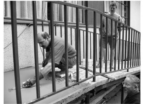
Greg lays down a smooth surface while mixers Gary and Arnie look on
